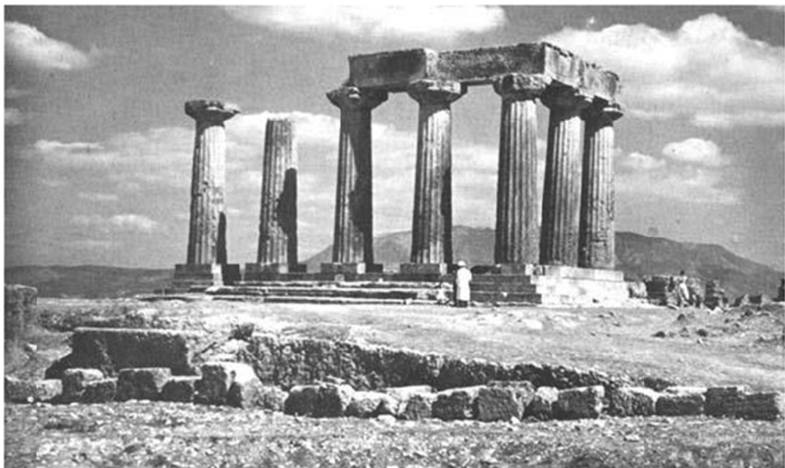
Doric columns of the archaic Temple of Apollo (6th cent. B.C.). Seven of the original thirty-eight columns survive, 24 ft. (7 m.) tall and 6 ft. (2 m.) in diameter. (W. S. LaSor)
