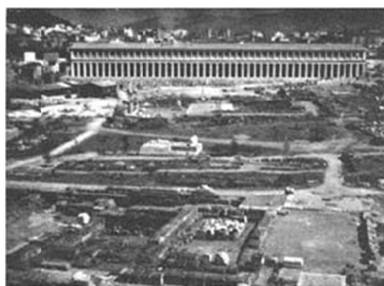
Ruins of the Hellenistic agora at Athens. The stoa of Attalos II (top, reconstructed) contained a row of twenty-one single-roomed shops on each of its two stories, each with a double colonnade. (W. S. LaSor)
