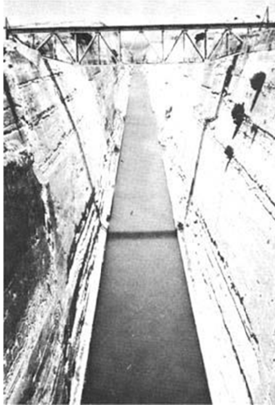
Corinth Canal, connecting the Ionian Sea and the Aegean, a distance of 3.5 mi. (5.6 km.). Constructed in 1881–1893, it follows the route planned and begun by Nero in A.D. 66. (B. Van Elderen)
