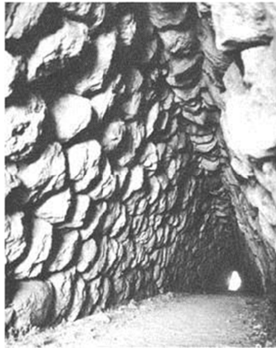
Postern tunnel with corbeled arch at Boghazköy (Hittite Hattusas) (B. K. Condit) 位于波格斯凯 (Boghazköy, 赫人都城哈图沙) 的带有突拱的后门隧道。(B. K. Condit)
